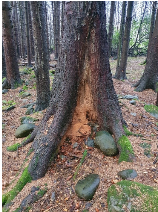
Figure 10: Decay at the base of a Sitka Spruce in the Dark Wood as a direct result of fire damage.
